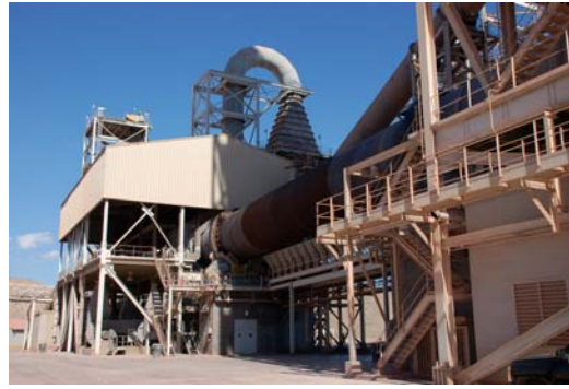
Cement Rotary Kiln, Clarkdale AZ
