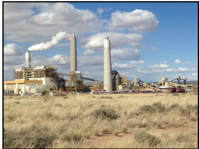
Coronado Generating Station
