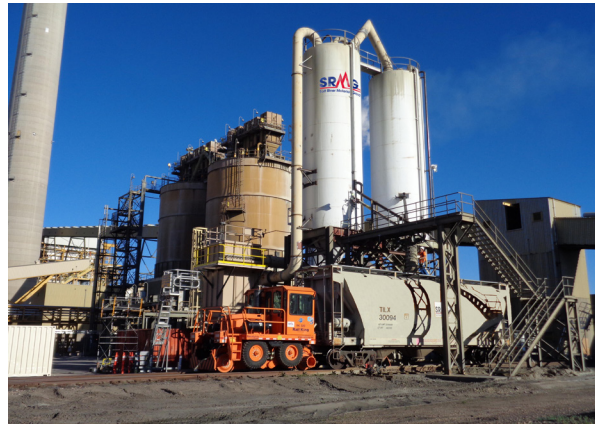
Coronado Generating Station Fly Ash Facility
