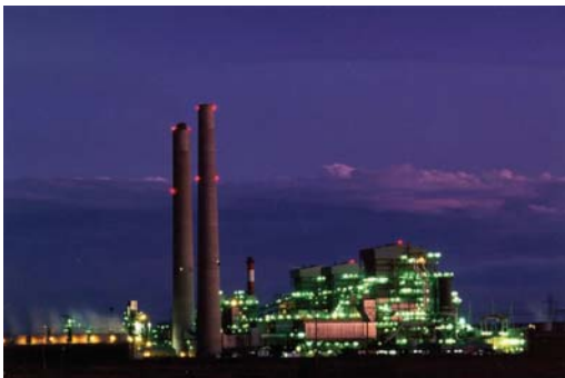
Cholla Power Plant
