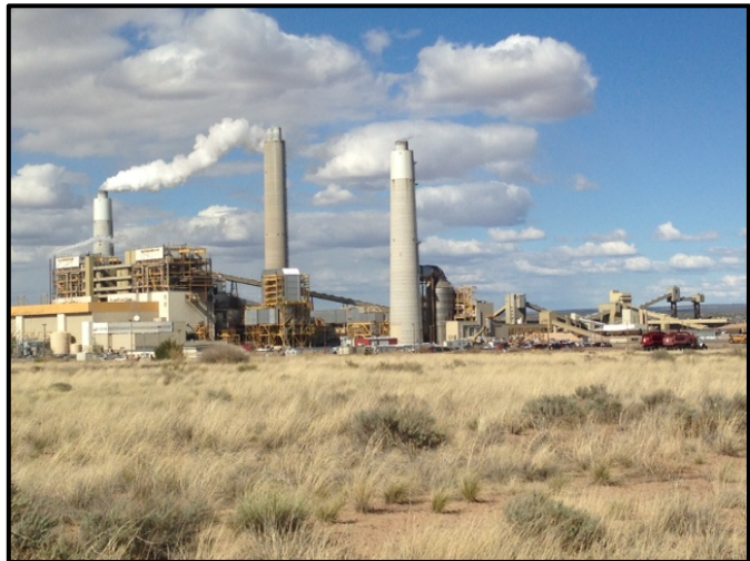
Coronado Generating Station, St. Johns AZ
